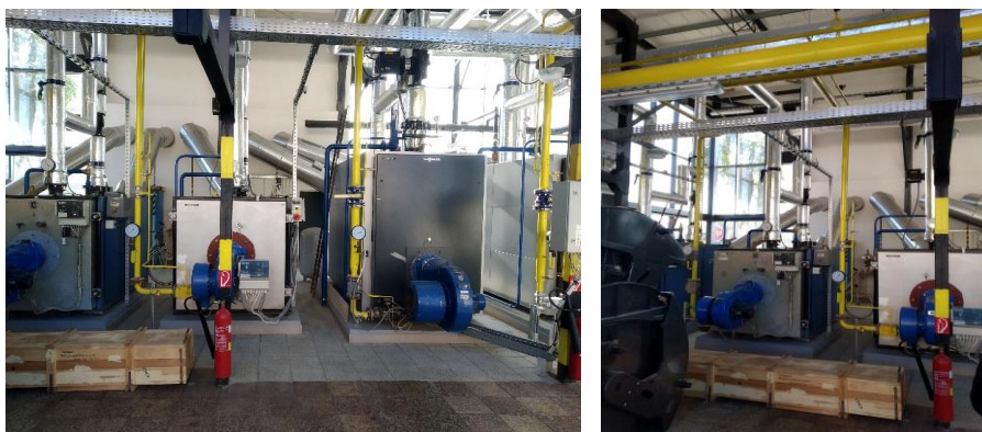
Fig. 4 View on the hot water boilers on natural gas (NG).
