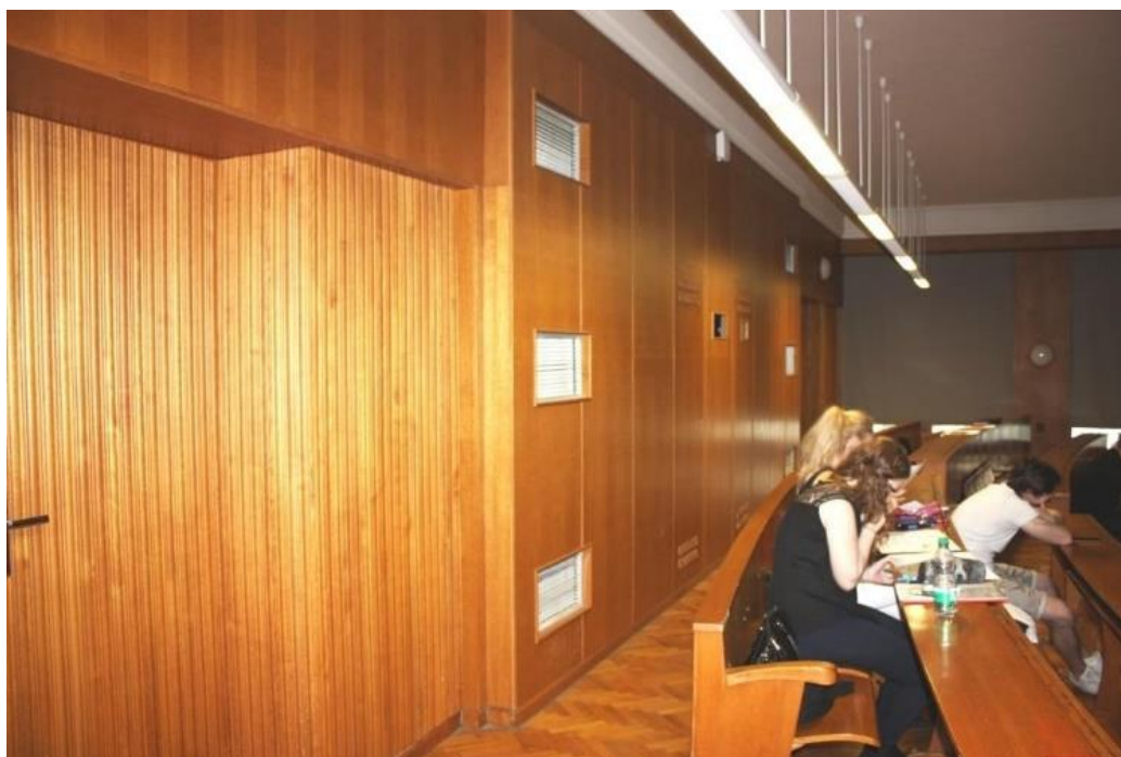
Fig. 2 Large lecture hall with the vents for extract air
