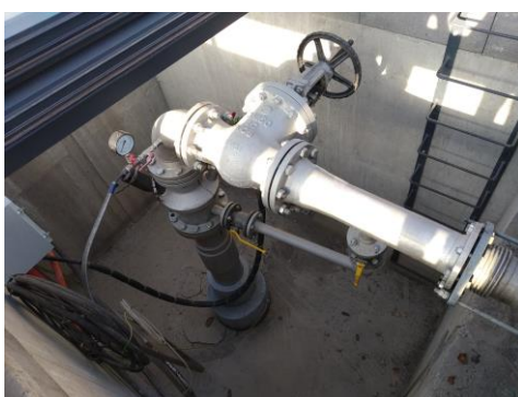
Fig. 1 Borehole head of well VM-1
