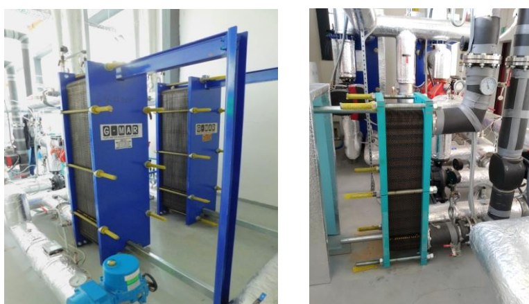
Fig. 3 Plate heat exchangers VT1 and VT2 and another PHE.
