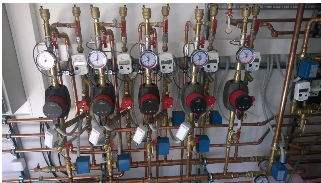
Fig. 3 Distributor and collector with measuring instruments on the heat transfer side [Author: Matej Kubica]
