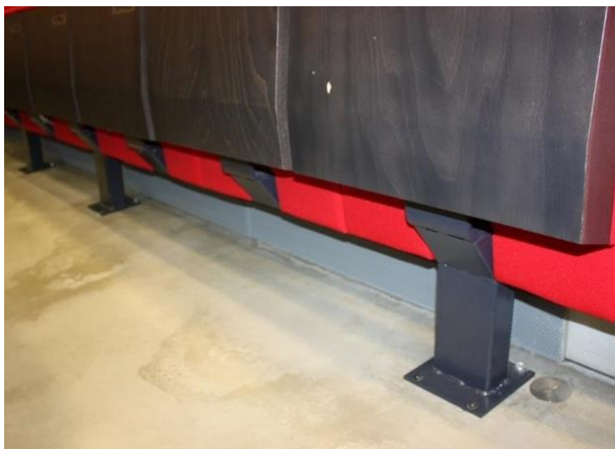
Fig. 2 Rectangular continuous vents for supply air in the stepped floor
